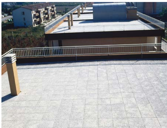
Tetto piano pedonabile
